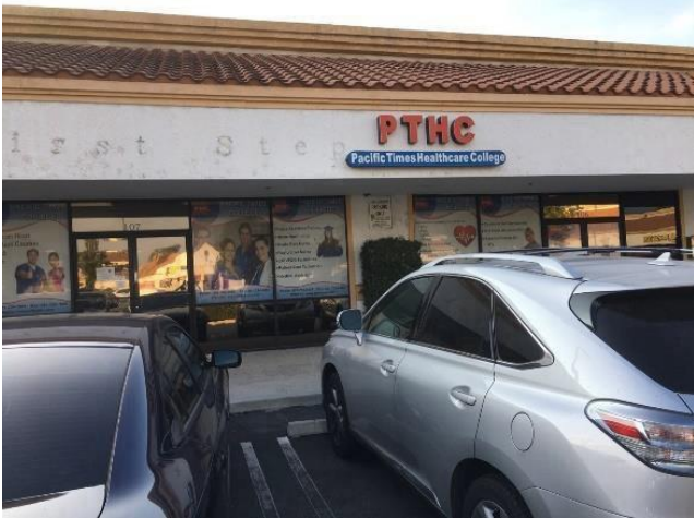
Front of Building
