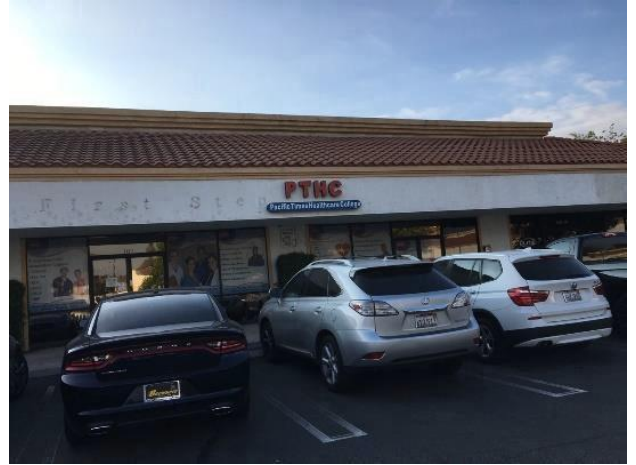
Front of Building
